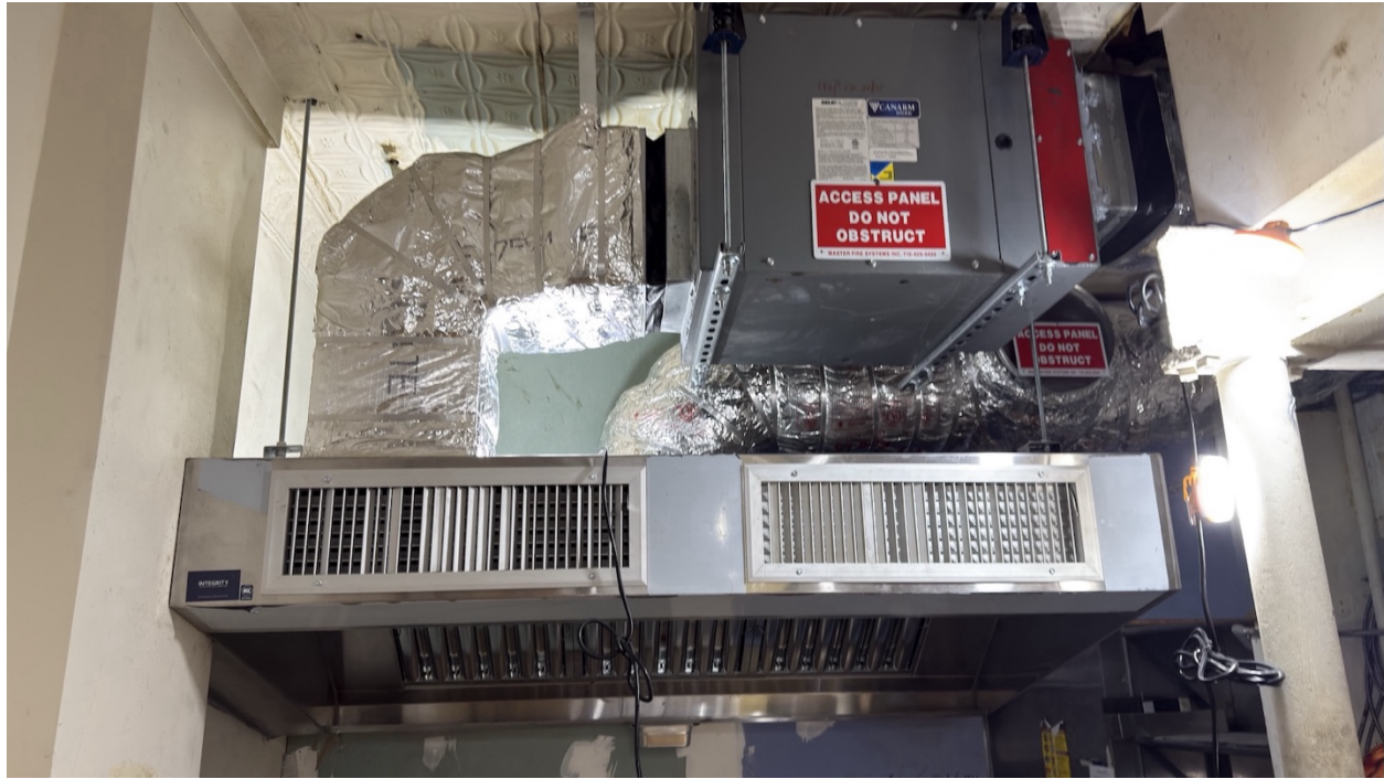
Photo Credit: Master Fire Canarm In-Line Blower : Brings fresh air from outside into the kitchen through the make-up air system.
